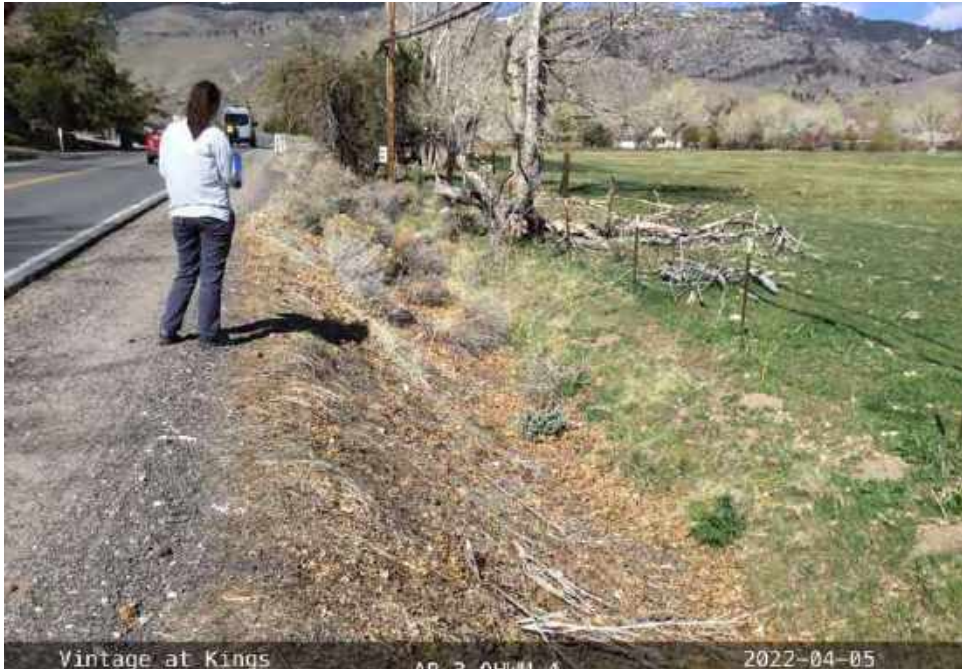
Photo 9. OHWM-4: AR-3 excavated roadside ditch at eastern end when some overland flow from irrigated pasture may intermittently be entering ditch. View looking west.
