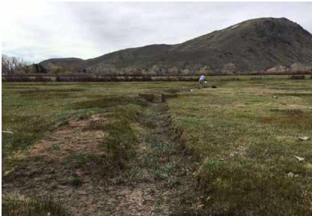
Photo 12. AR-4a: Southern end of AR-4 excavated irrigation ditch. Old irrigation ditch capturing sheet flow across pasture. Small weir visible in picture no longer operating. View looking south.
