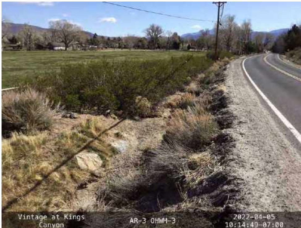
Photo 8. OHWM-3: AR-3 excavated roadside ditch capturing storm water from road. When present, water flow from west to east into storm drain at southeast corner of Survey Area. View looking east.
