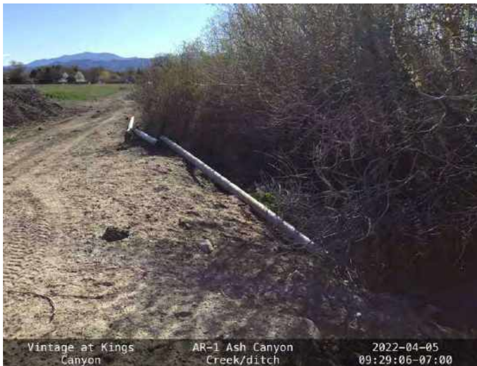
Photo 4. Overview of Ash Canyon Creek (AR-1). View looking east on north bank.
