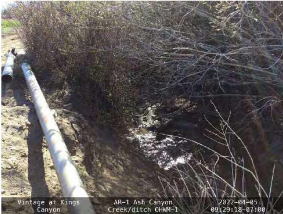
Photo 5. OHWM-1: picture showing approximately 2-4 inches of water in Ash Canyon Creek (AR-1). Exposed/partially excavated left bank with disconnected irrigation line. View looking southeast.
