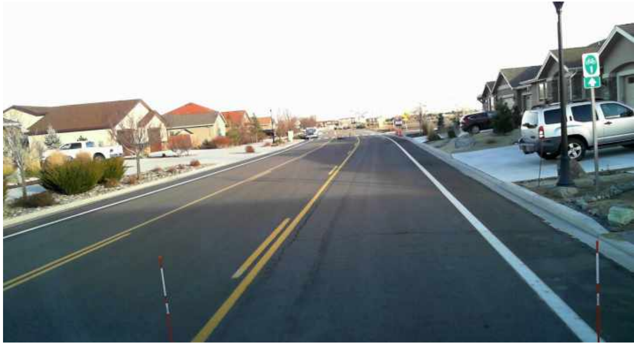
Figure 3. Pavement in Satisfactory condition category (PCI 85-71).
