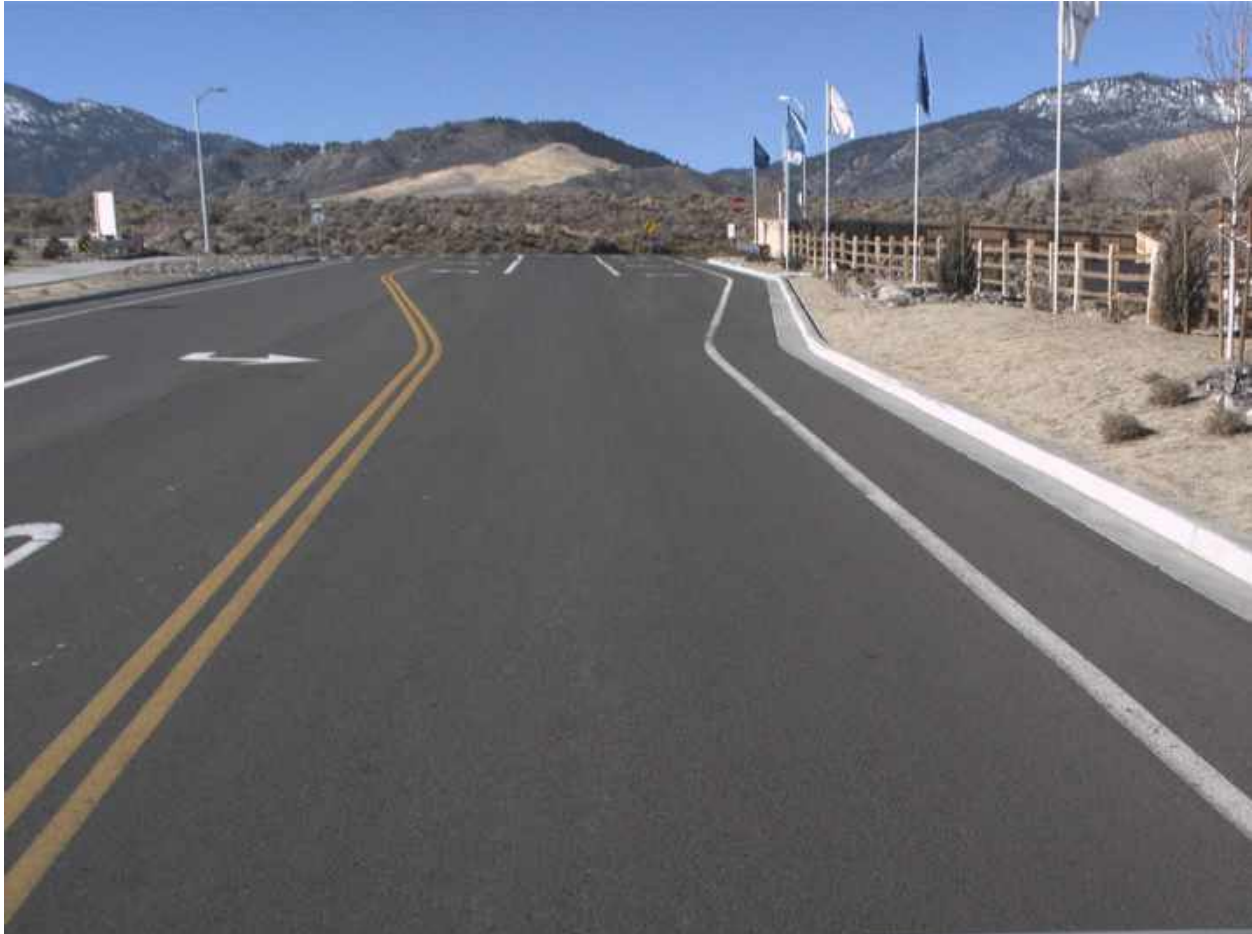
Figure 2. Pavement in Good condition category (PCI 100-86).
